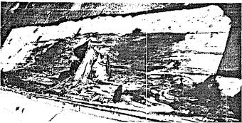
Figure 15. (a) A regular cleaning schedule would have eliminated the plant growth and leaf build-up in this gutter, which, if not removed, will result in serious damage to roof sheathing and structure (b). Photos: (a) Paul K. Williams, and (b) Walter S. Marder. AIA.
