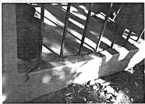
4.16 Rusted rails and spalled concrete at front porch NCO Type B.
