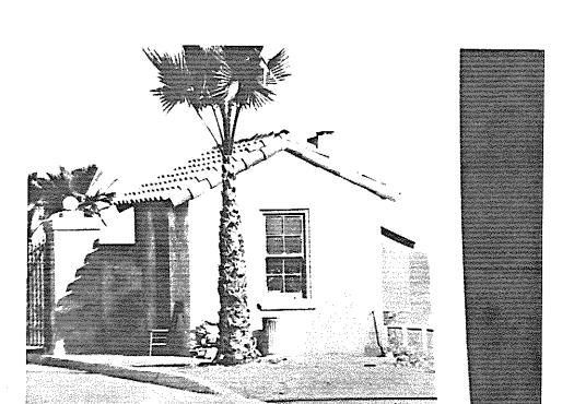
9.17 View showing original double-hung four-light wooden windows and original light fixtures.
