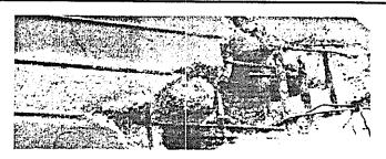
Fig. 13b. Upon removal of the deteriorated surface, a pocket of poorly mixed concrete (mostly sand and gravel) was easily chiseled out. The reinforcing rods were in good condition.
