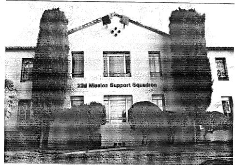
9.44 The facade retains a high degree of historic integrity, including original steel casements.
